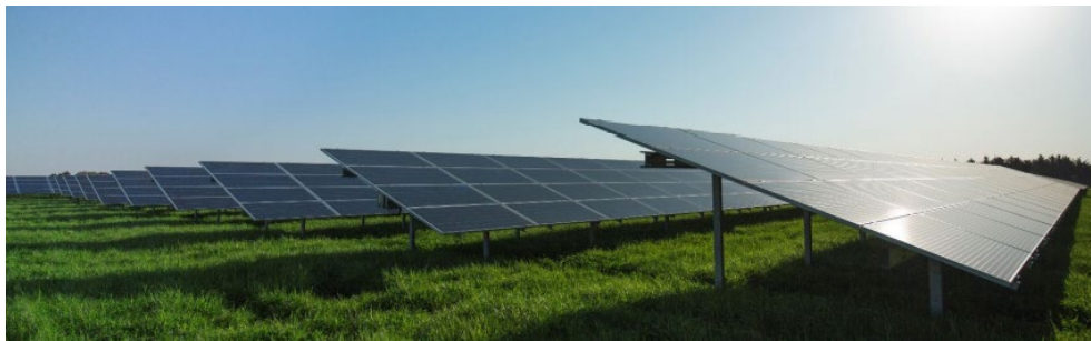
Figur 1-4 Princip for opstilling af solcellepaneler.
