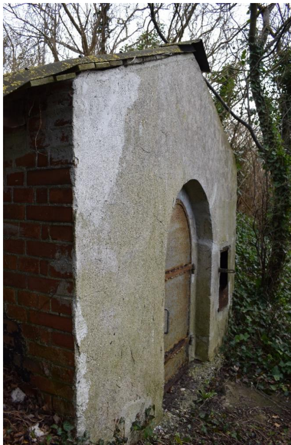
Krudthus, gavl mod nord
