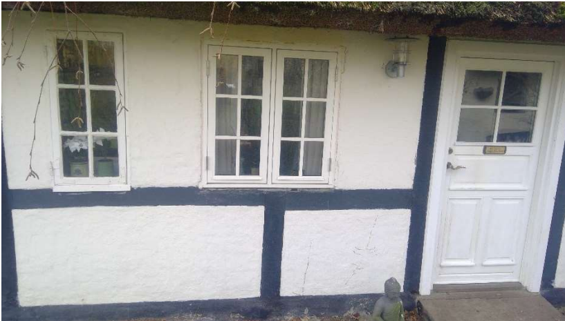
Facade mod have
